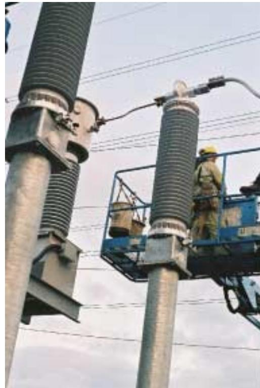
Fig. 1. A 138 kV NXVCT system being installed at Hydro Quebec's Rolls Royce substation near Montreal, Quebec, Canada
